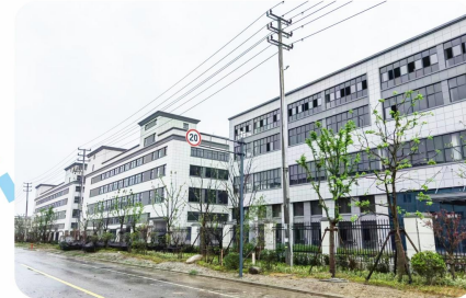
High-tech zone site
